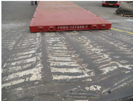
Fig. 3 – Operation of loading / unloading INCORRECT
